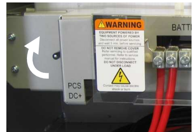
Figure 14: Battery breaker disconnect turn ON.
